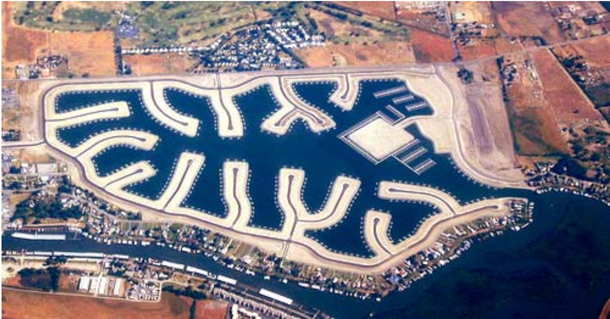
Delta Coves, a partially developed subdivision on Bethel Island without water to the fire hydrants
