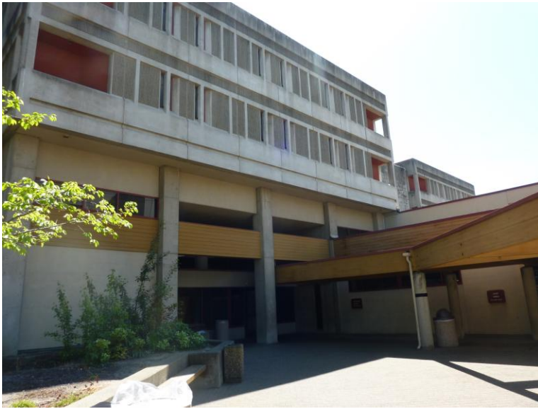
The Martinez Detention Facility in Downtown Martinez
