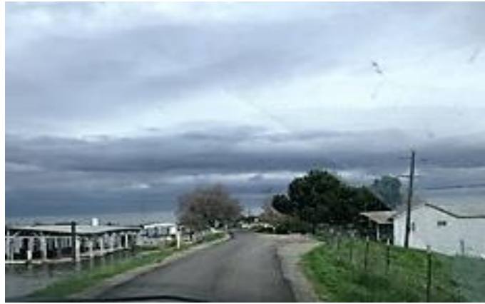
GJ photos: Pictures of levee crowns
